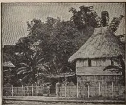
FIG. 374. A native house in Manila in the Philippines built of bamboo and straw. It is very suitable to a hot, damp climate, where the people are only half-civilized and have very few wants.
